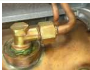
A fitting that uses sealant to seal it.
